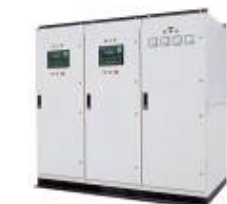
DSE50 Parallel Control Panel system
